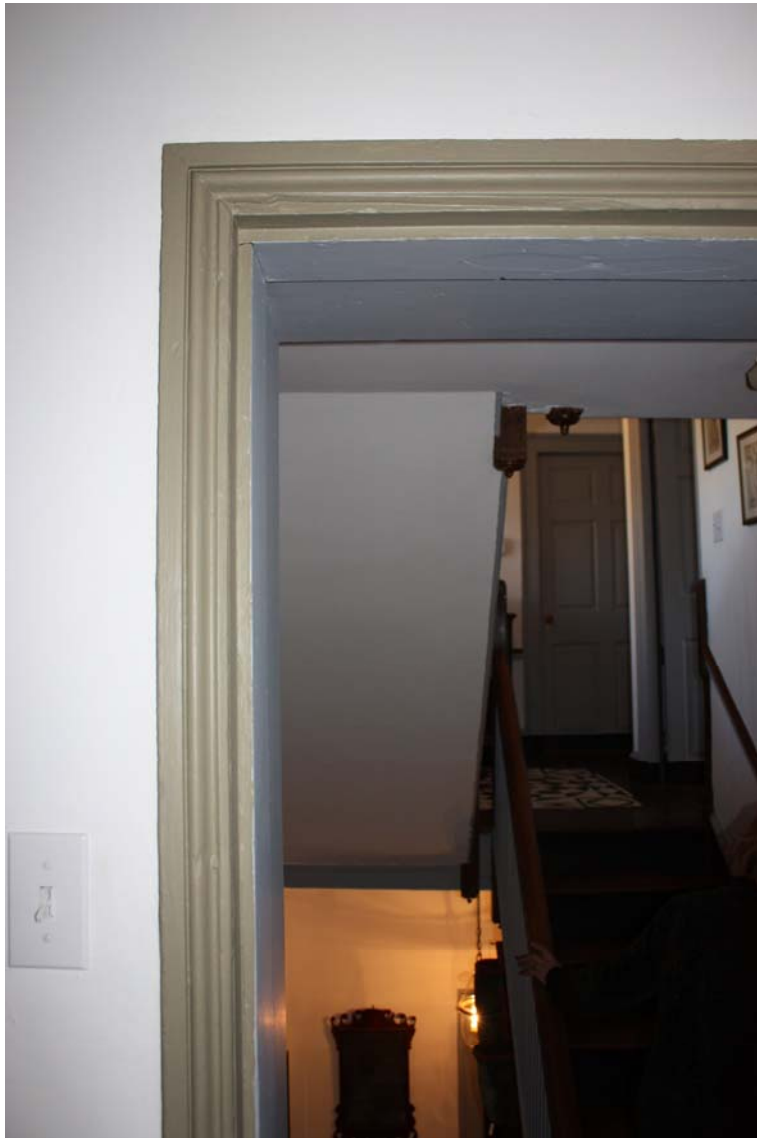
Figure : Second period molding profile; second floor, bedchamber in west wing, over original kitchen (now dining room); same as in bedchamber above in third floor, and in doorway between original and current kitchen (ell).
