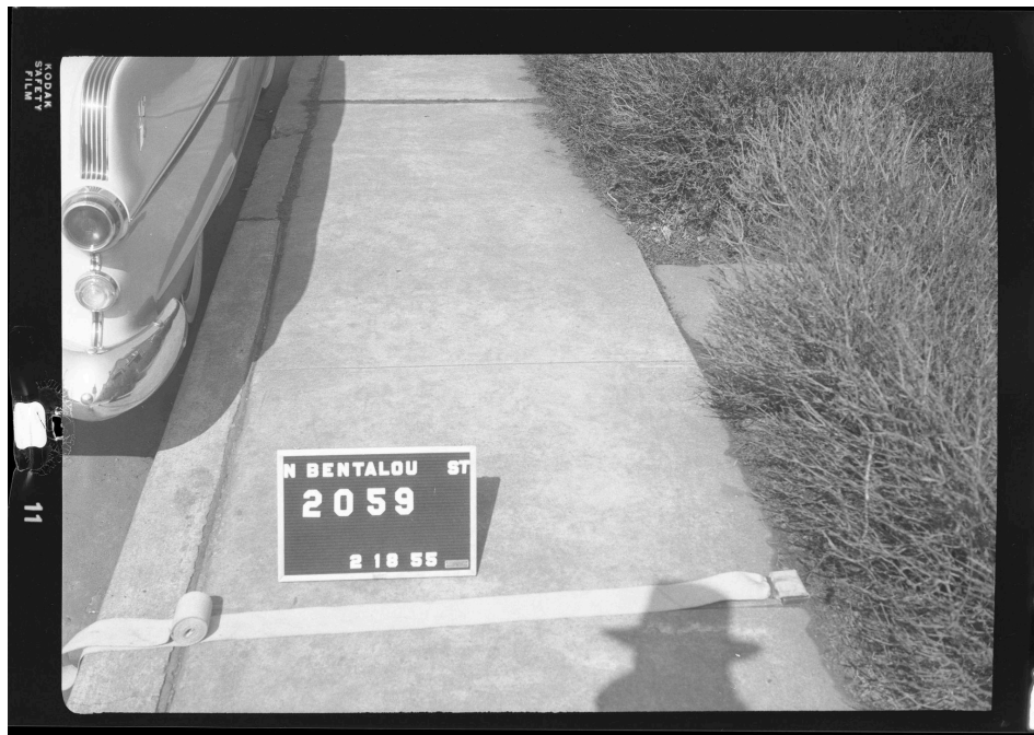
One of thousands of negatives acquired from the Department of Public Works, capturing glimpses of Baltimore City sidewalks: 2059 N. Bentalou Street, February 18, 1955
