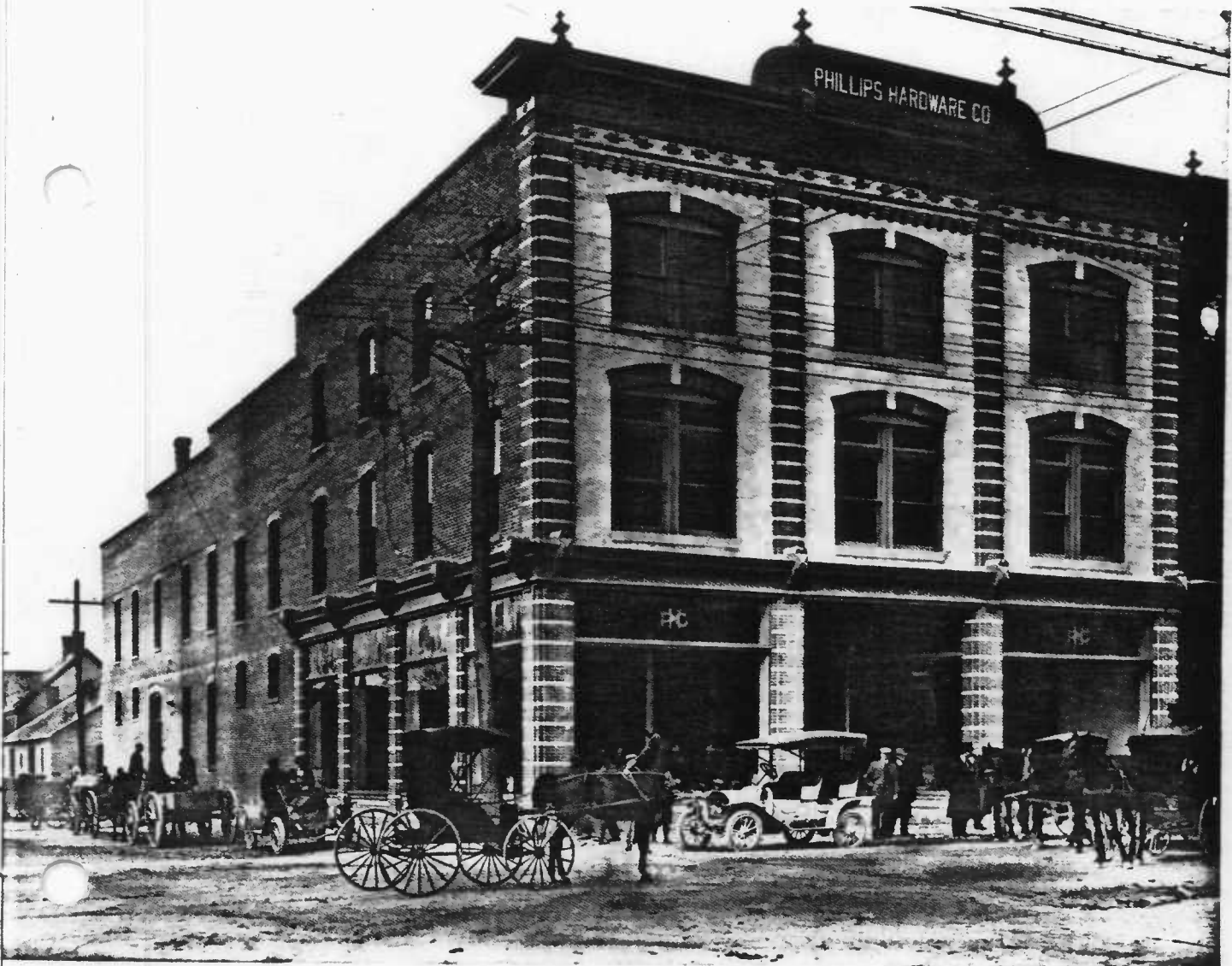
After the fire of July 31, 1910, the Phillips Hardware Company purchased the lot where the home of Mary E. Winterbottom had burned; on this site, opposite their former location, the company erected this modern building for its hardware business. Photograph circa 1911-13 by J. Watson Thompson; courtesy of Morley Jull collection
