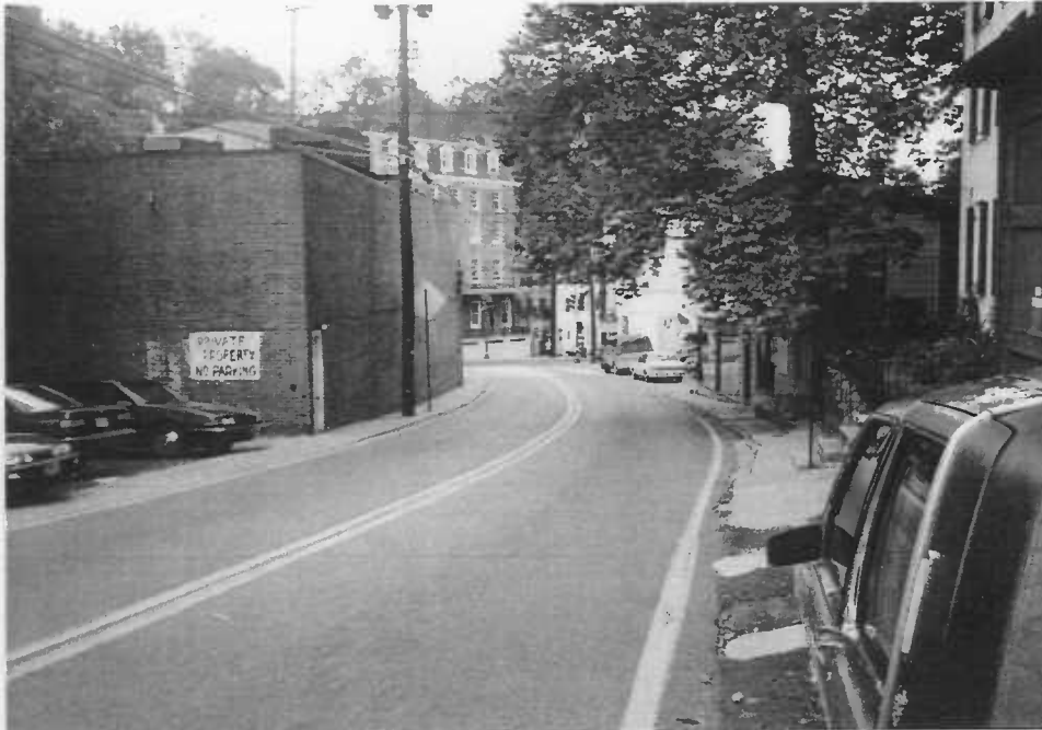
NO. 2 - SOUTH APPROACH
