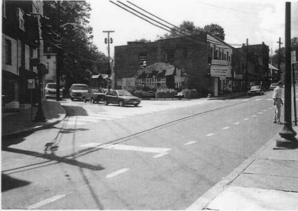
NO. 1 - NORTH APPROACH
