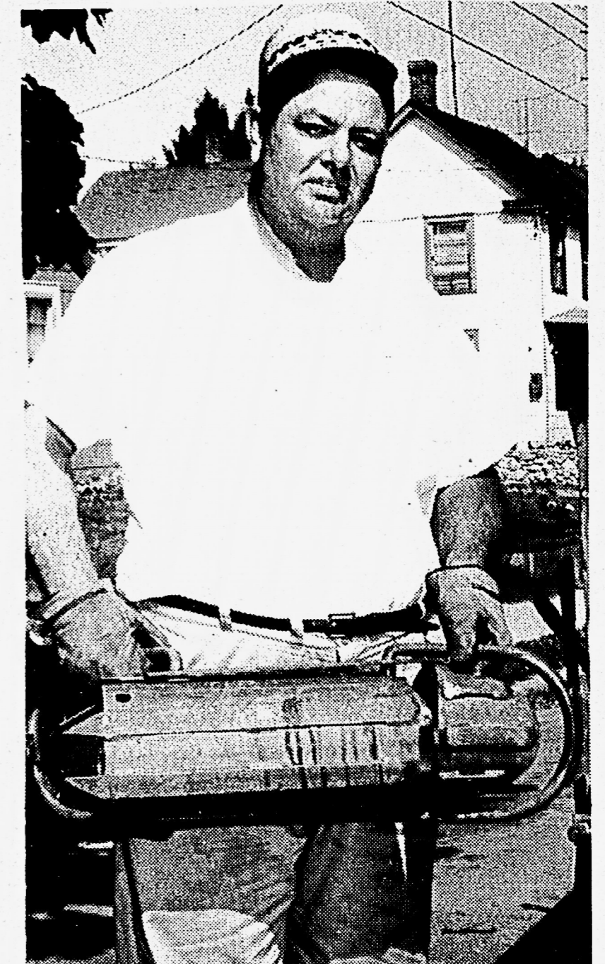
Medford C. Capel, assistant engineer of the Chestertown Utilities Commission is shown with bucket used in new O'Brien Sewer Cleaner.
