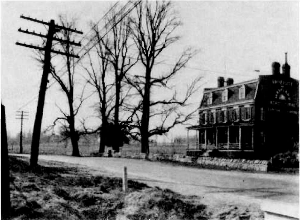
FIGURE 11. The Rossborough before the 1938 Renovation, photograph by W. F. Kellerman, 1926. University of Maryland, Special Collections and University Archives, Phi Mu Fraternity records, Initiation Paper 1923–1945, Box 5, Folder 4.0
