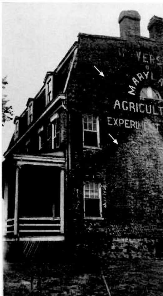
FIGURE 13. This image shows the ghost line of the wing and the former roof line, Anonymous, 1938. University of Maryland, Special Collections and University Archives, Work Projects Administration in Maryland records, 3358
