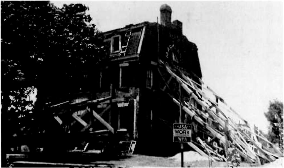
FIGURE 12. The walls of the Rossborough were heavily braced during the renovation, Anonymous, 1938. University of Maryland, Special Collections and University Archives, Work Projects Administration in Maryland records, 3358
