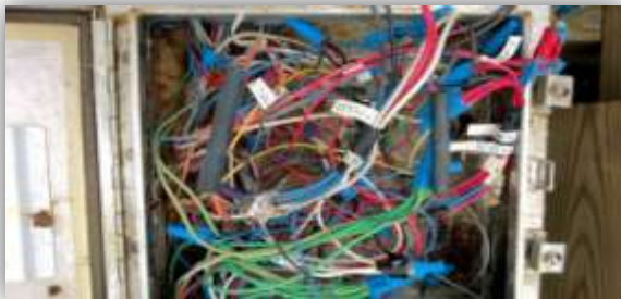
Fuel pier electrical box damage.
