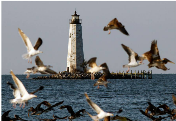
Restoring the Chesapeake Bay is an important commitment for Howard County and this Plan.
