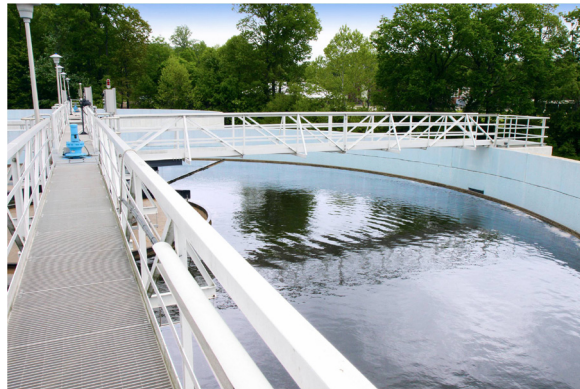
State-of-the-art technology and facilities are hallmarks of Howard County's wastewater treatment.
