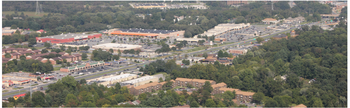
The Route 40 Design Guidelines and Streetscape Master Plan provide guidance for enhancing the corridor's function and aesthetic qualities.
