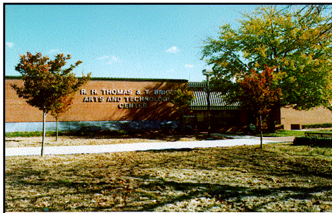
The Arts and Technology Building
