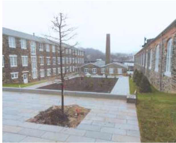
(Union Mill, located in the Hampden National Register Historic District in Baltimore City, was rehabilitated by Seawall Development Company using Sustainable Communities Tax Credits.
