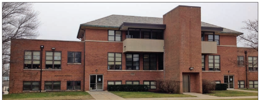
Bledsoe Building, 1953, last remaining building on Overlea Campus from the Colored School for the Deaf. It is scheduled to be razed in the near future.
