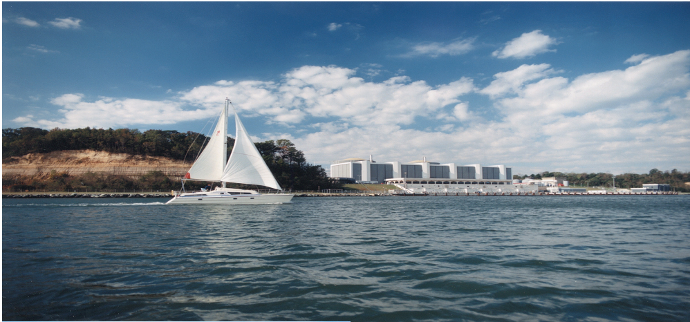
Calvert Cliffs Nuclear Power Plant
