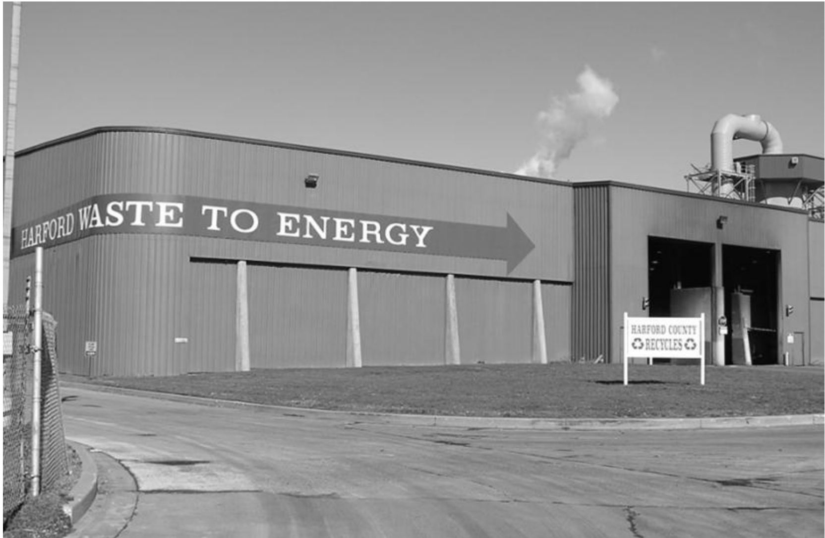
Waste to Energy Plant
