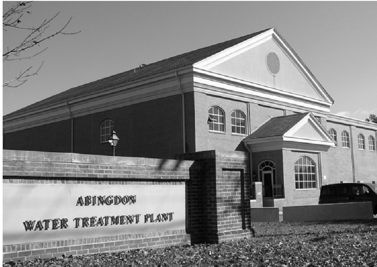
Abingdon Water Treatment Plant
