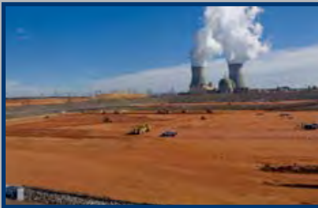
Above: Compacting backfill for Unit 4 with Plant Vogtle Units 1 and 2, December 2, 2010. SOURCE: 2010 Southern Company, Inc.
