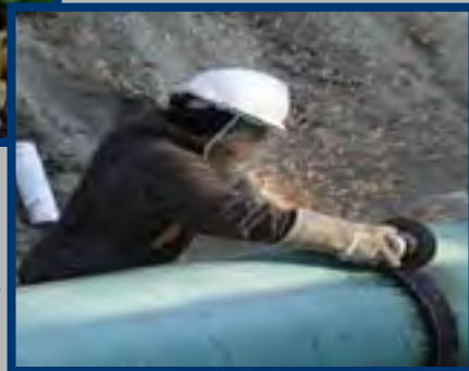
Right: Denbury's Green Pipeline construction. SOURCE: Denbury Resources, Inc.
