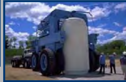
Below: Mobile transporter unit moves spent fuel dry storage cask for placement on a concrete pad. SOURCE: Nuclear Power Plant Spent Fuel Storage Systems
