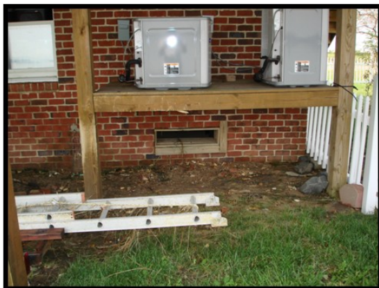
A homeowner elevates critical HVAC components for their home, mitigating flood damage
