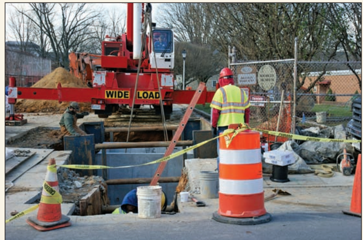
Water vault is gently lowered into position.
