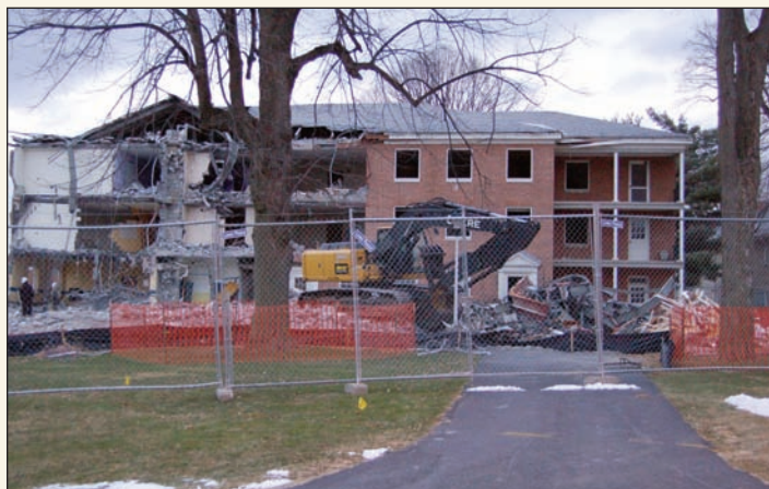
Demolition of Barry Hall in progress
