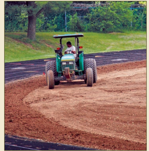
Dead grass is removed and new soil is spread over the field.
