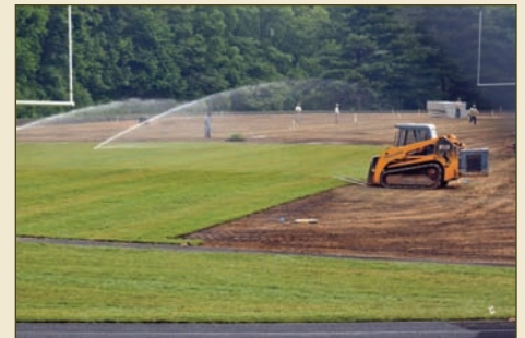
Use of irrigation system to water the field begins even before re-sodding is complete.
