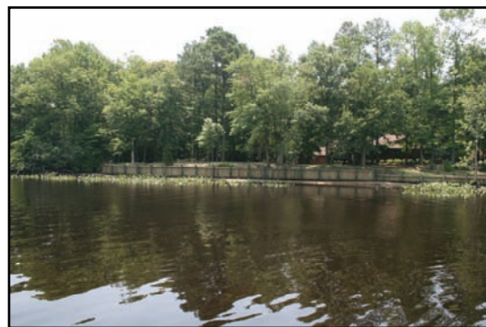
Hardened shoreline witnessed on the river tour
