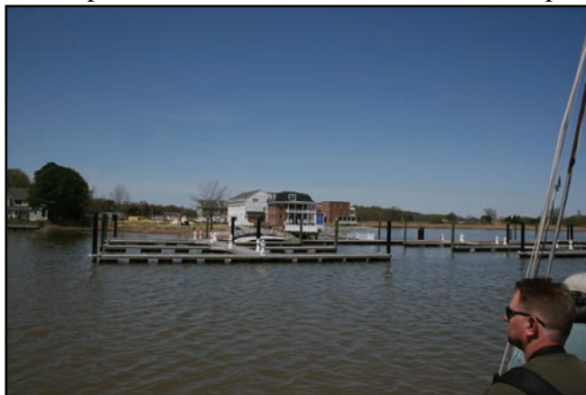
Chester River Landing under construction, April 16, 2008
