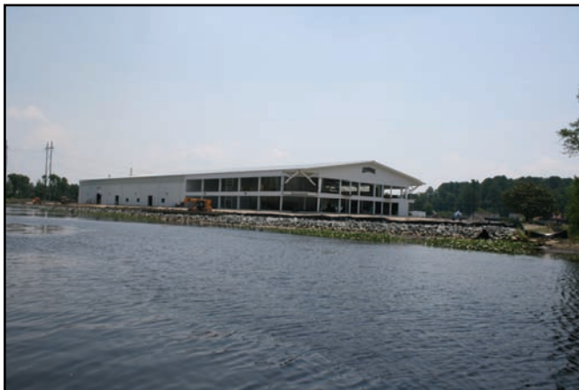
Riprap shoreline seen on the boat tour
