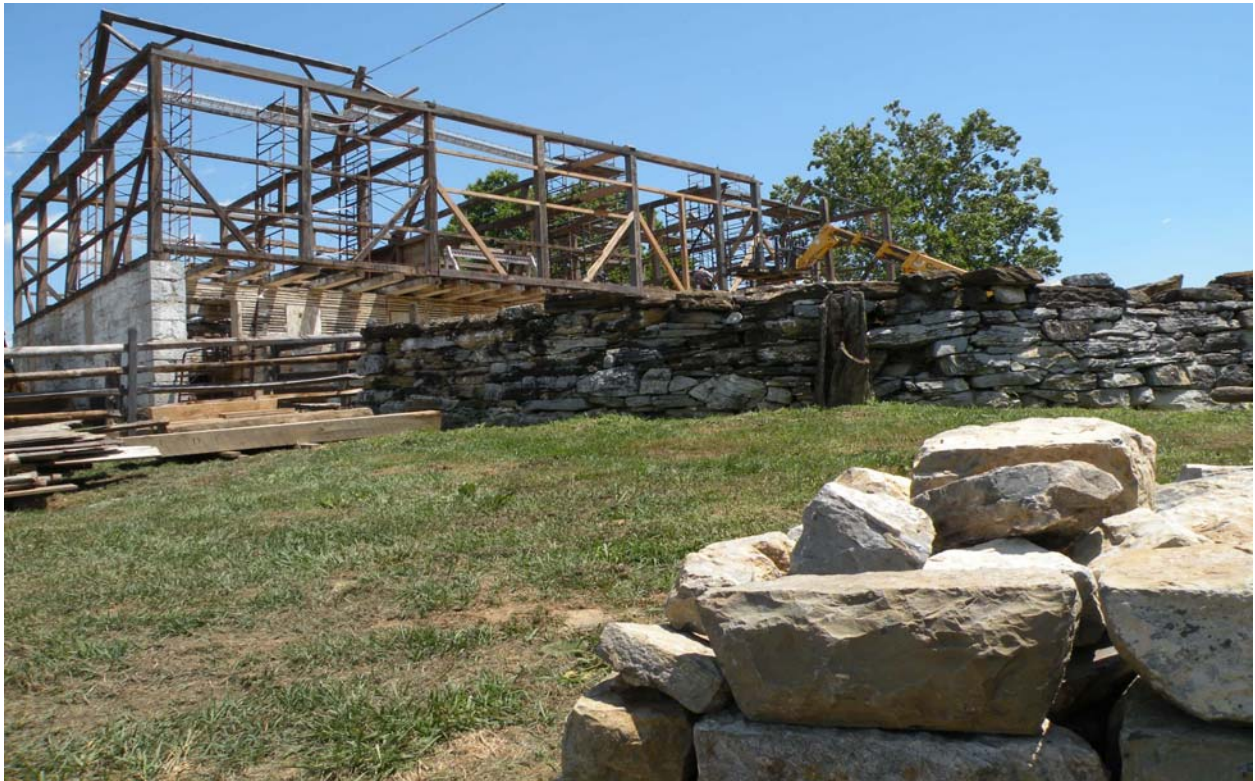
Original MCI-H stones (foreground), quarried on-site in the 1930s, stand ready to restore the Poffenberger barn and stone wall out front at Antietam National Battlefield.
