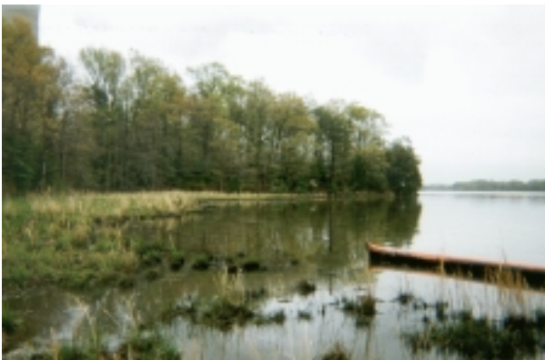
Containment boom placed at the mouth of Swanson Creek to control the migration of spilled oil into the Patuxent River. Chalk Point Power Plant is in the left background.
