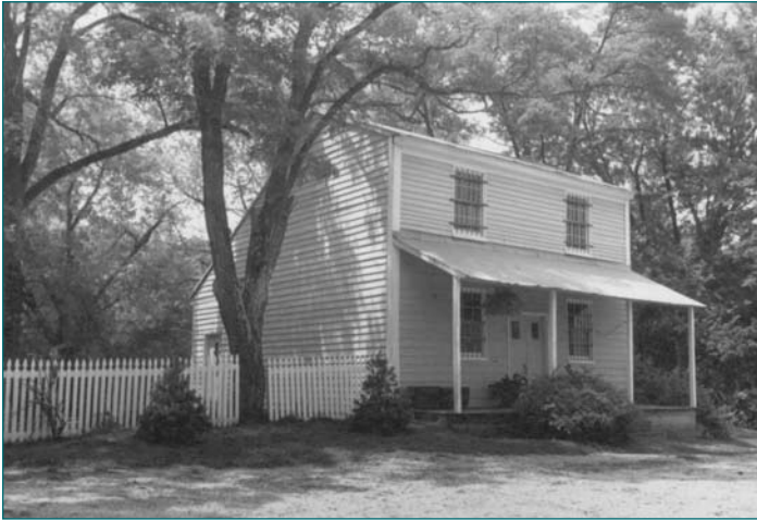
86A-027-11 Coffren Store (NR) 10007 Croom Road Croom
