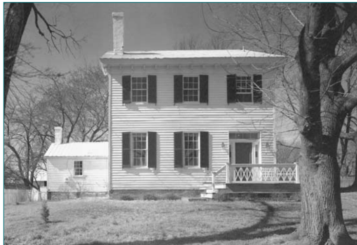
86A-027-10 Coffren House (NR) 10007 Croom Road Croom
