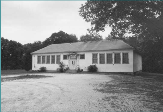
87B-034 Woodville School 21500 Aquasco Road Aquasco
