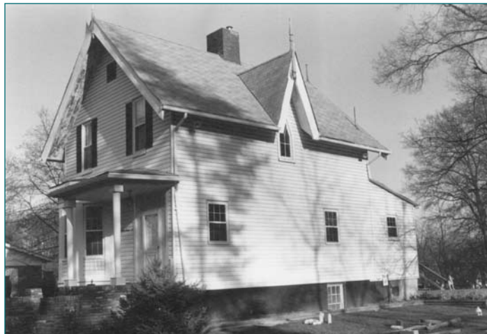
70-053-12 Seabrook Cottage 9425 Dubarry Street Seabrook
