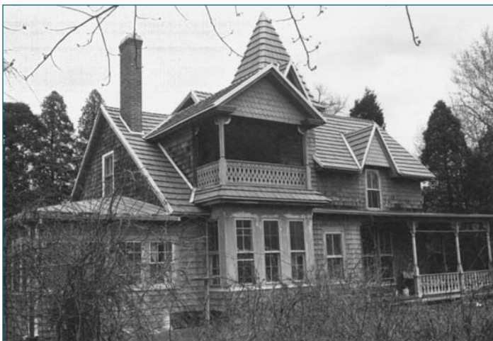
71A-003 Ingersoll House 9006 Laurel-Bowie Road Bowie vicinity
