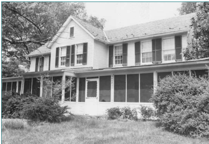
72-006 Carmody House 6808 Drylog Street Seat Pleasant vicinity
