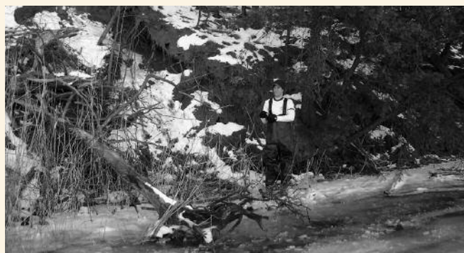
This heavily eroded cliff along Back Creek will be restored with funds provided through the Trust's Living Shoreline Grant Program.
