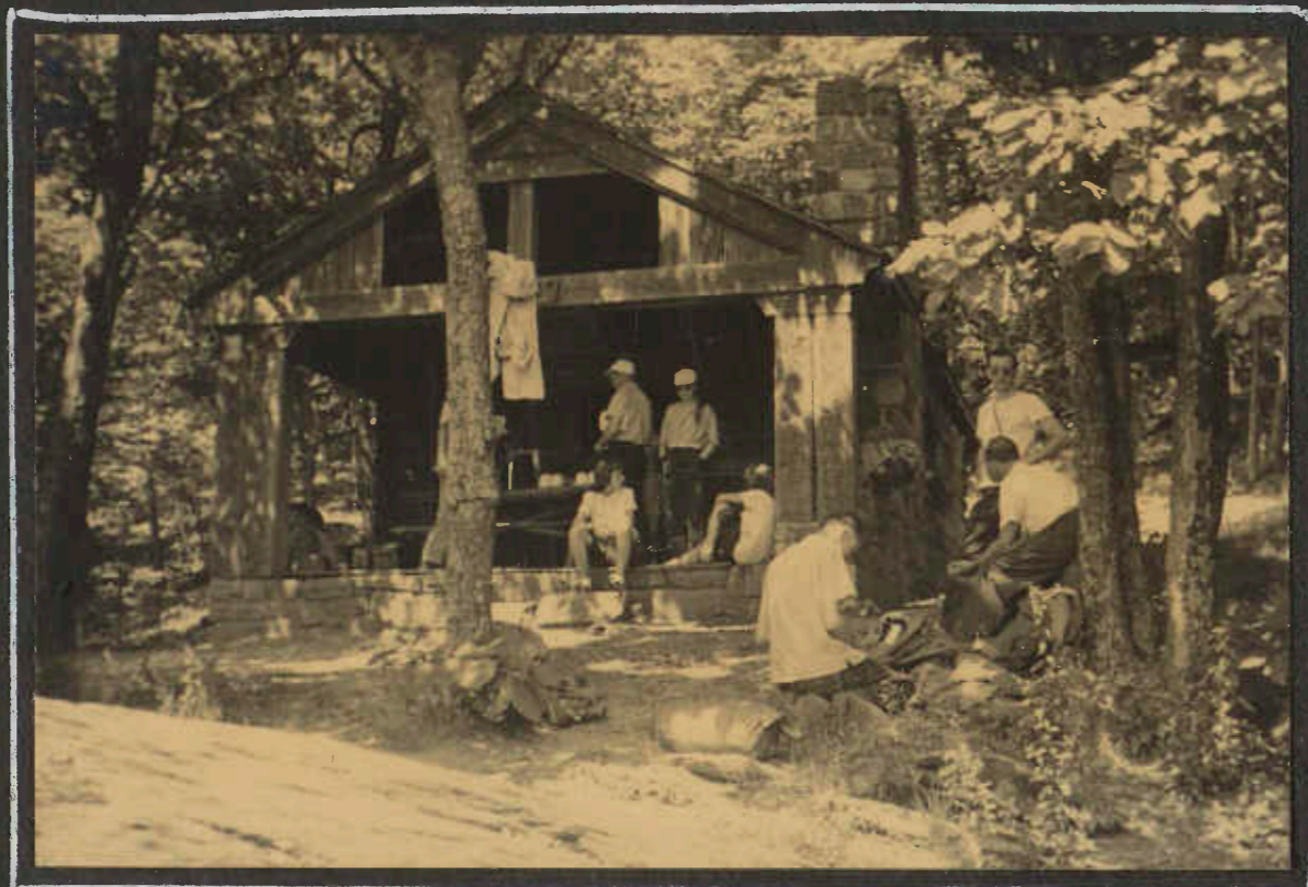
BASE CAMP - DOYLE RIVER SHELTER
