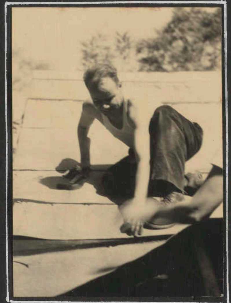
WINSLOW BECOMES ROOFER
