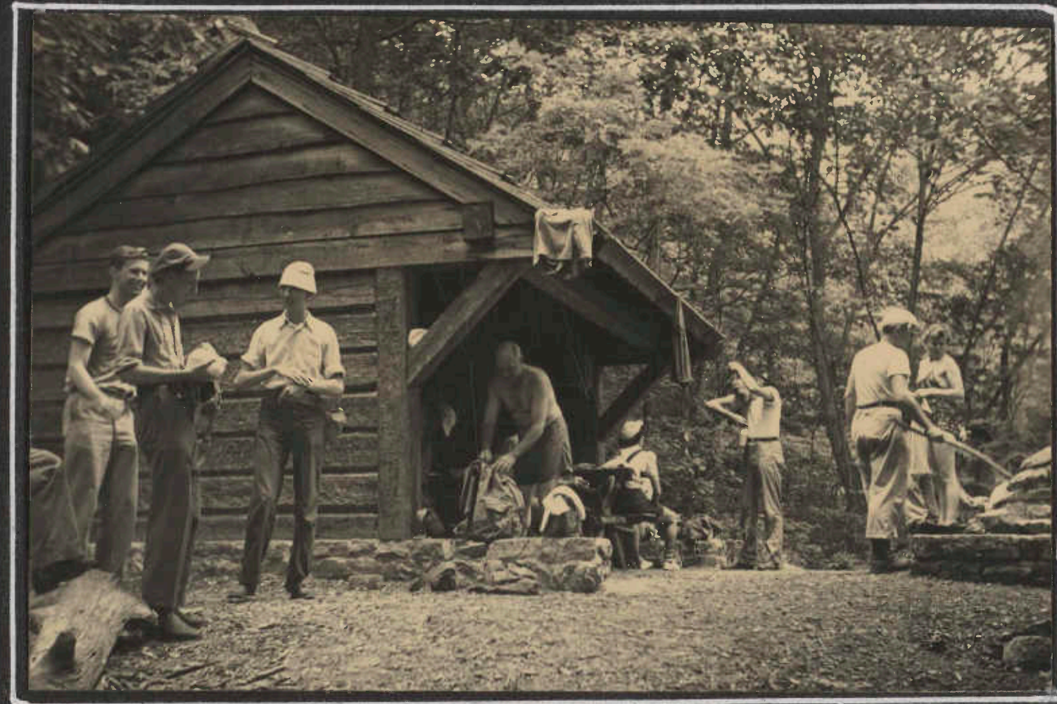
AT THE RIP RAP SHELTER
