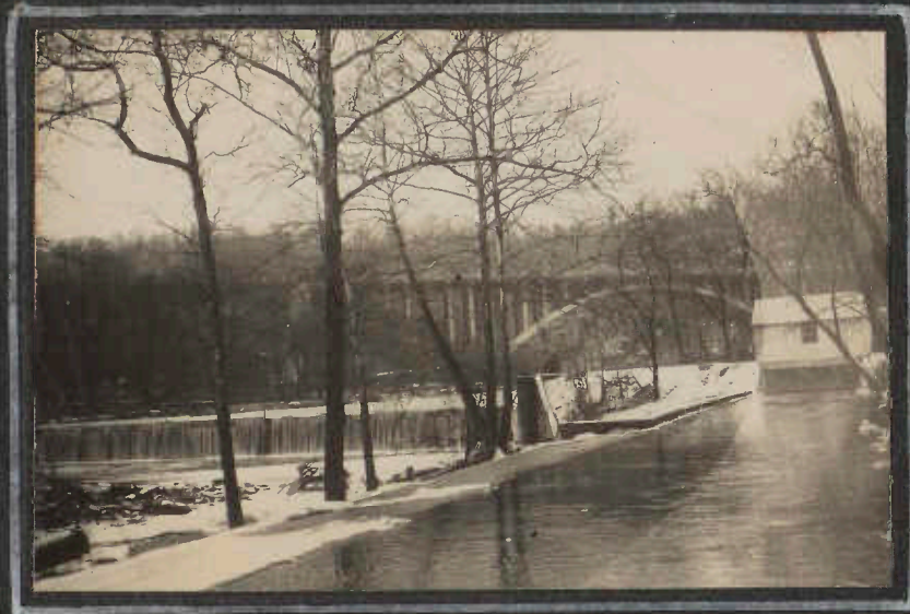
UNION DAM, THE MILL RACE, AND THE HIGHWAY BRIDGE (BYPASS 40)
