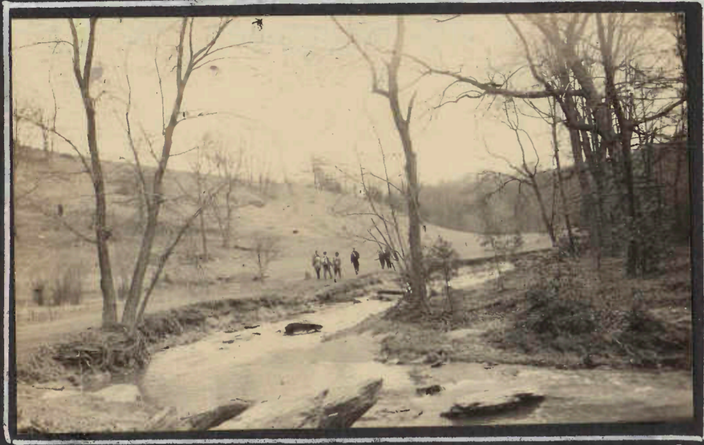
SECOND MINE BRANCH
