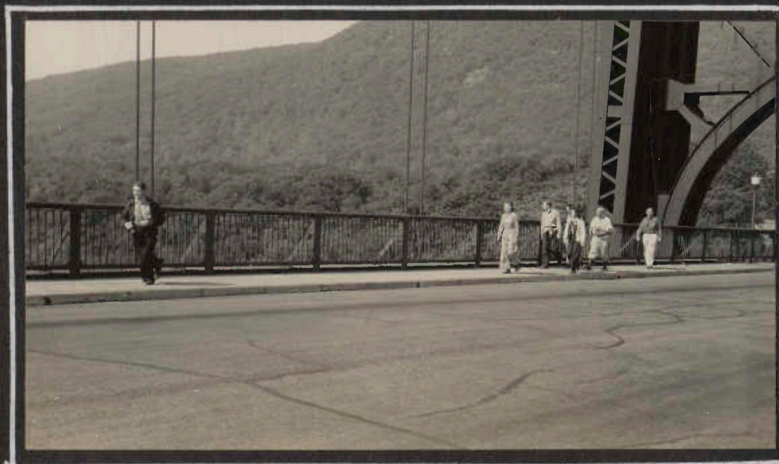
CROSSING BEAR MOUNTAIN BRIDGE - LOWEST POINT ON THE APPALACHIAN TRAIL. ORVILLE RUNNING AHEAD TO GET A PICTURE
