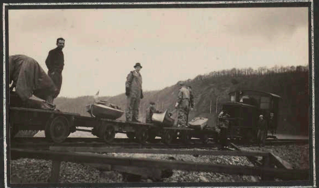
THE REASON FOR INCLUDING THE PICTURES IN THE ALBUM -- LAW REQUIRES THE POWER COMPANY - ON DUE NOTICE - TO HAUL BOATS AROUND THE DAM --- FREE NAVIGATION ON THE SUSQUEHANNA - AND HERE WE HAVE THE TRAIN ASSIGNED TO THE JOB ---
