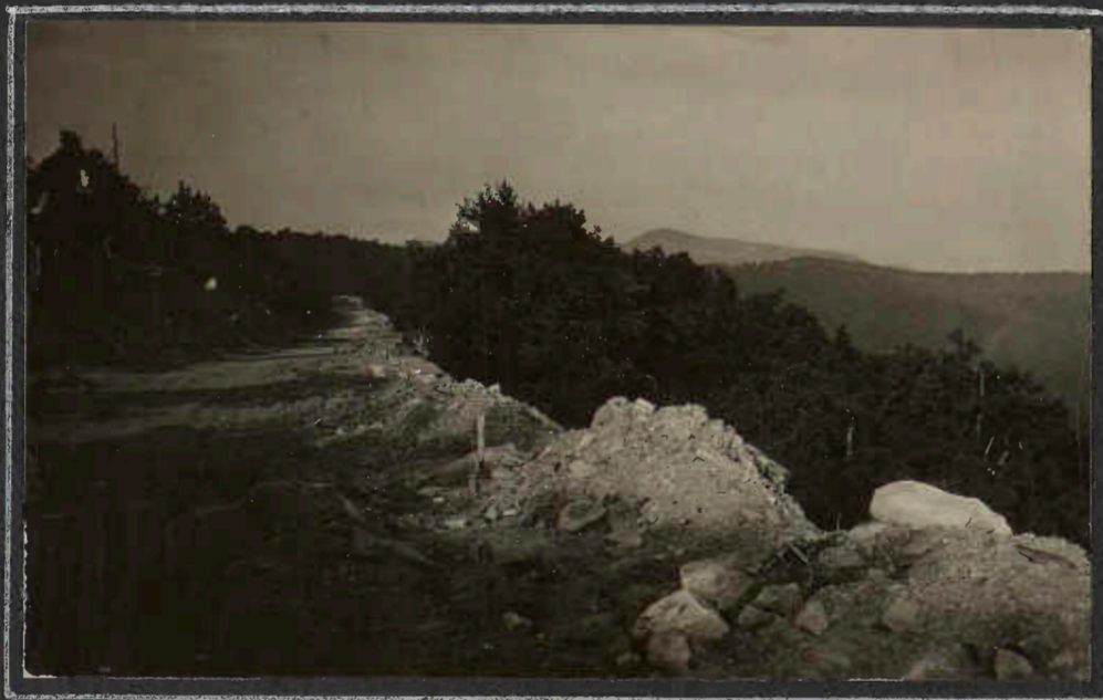
THE SKYLINE DRIVE UNDER CONSTRUCTION
