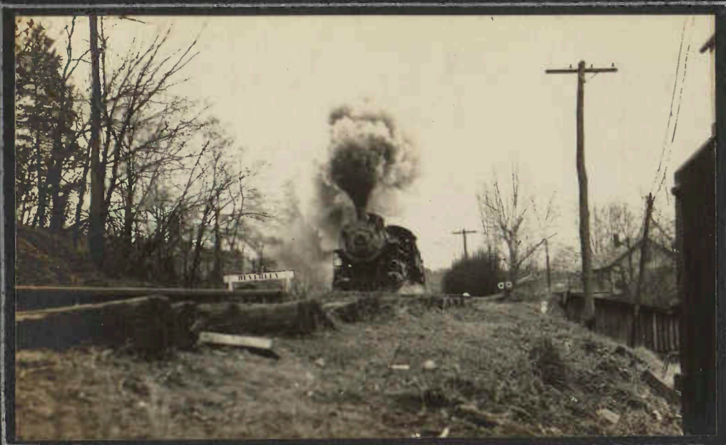
THERE'S A RAILROAD THRU THIS COUNTRY....
