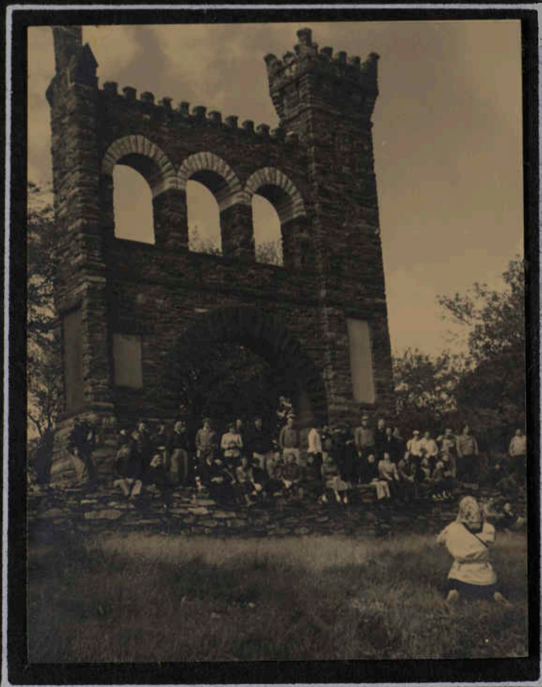
GROUP ASSEMBLES AT CRAMPTON GAP
