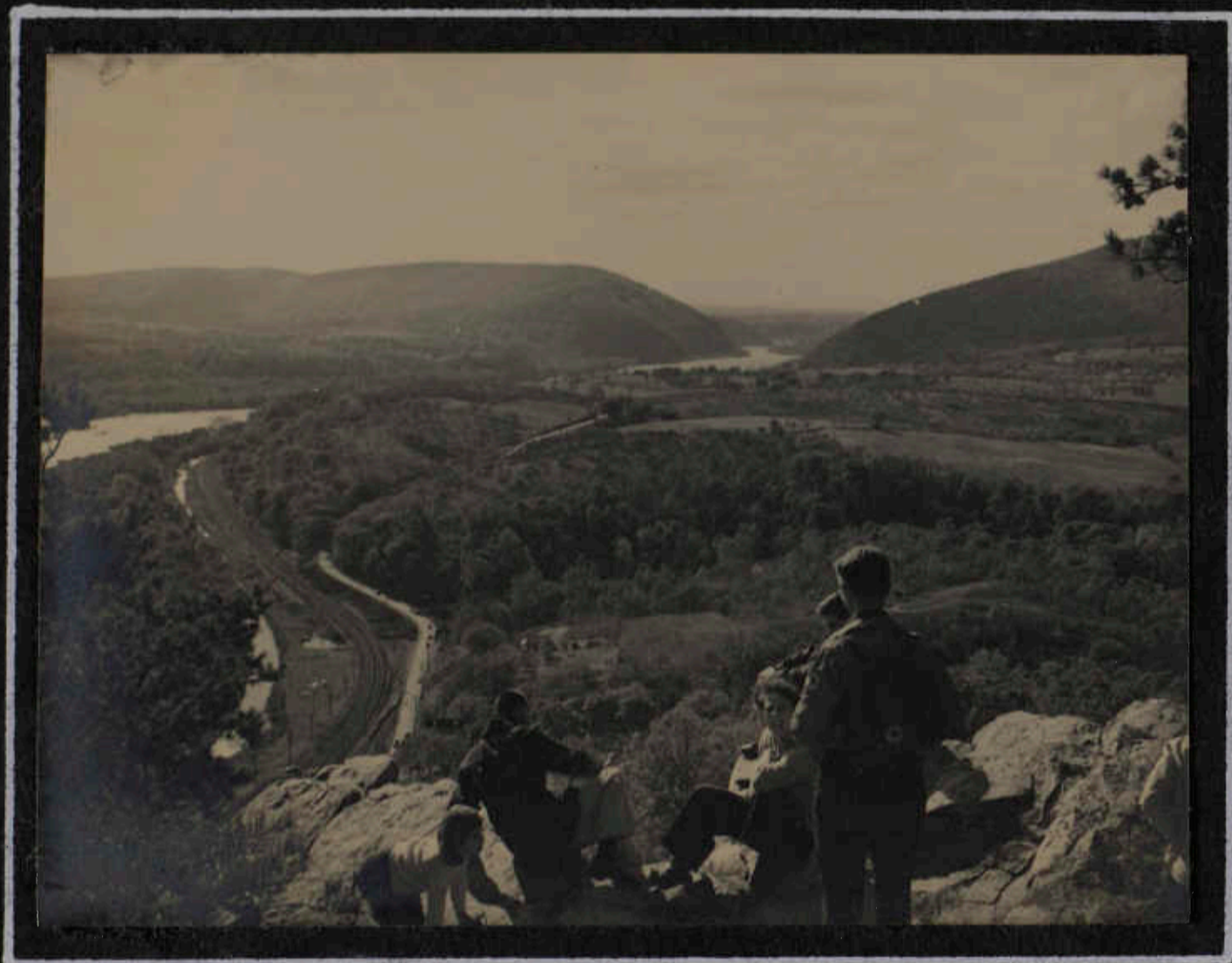
REST STOP ON WEVERTON CLIFFS Roessler
