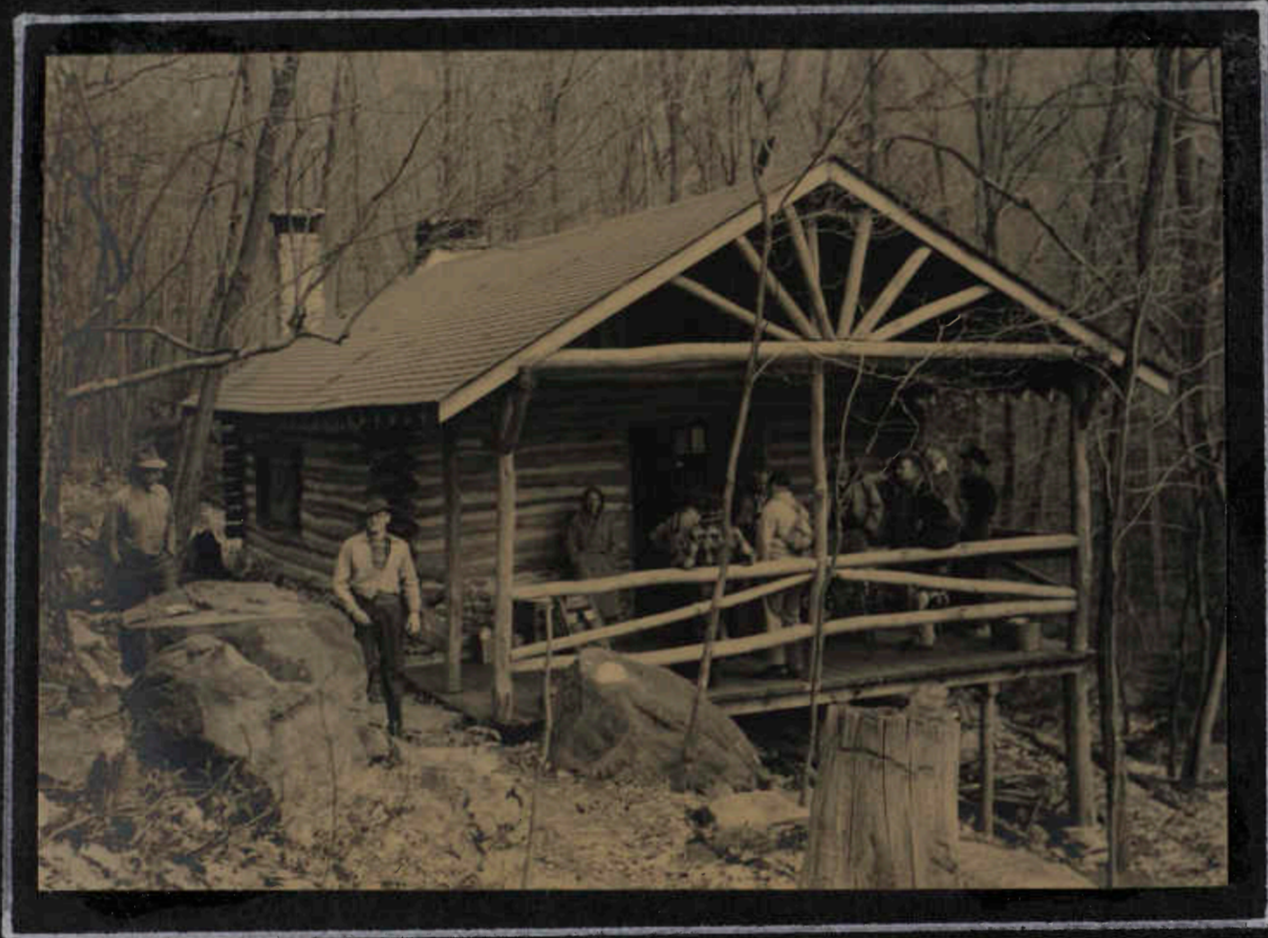
HERMITAGE SHELTER - THE STRUCTURAL ENGINEER'S NIGHTMARE.
