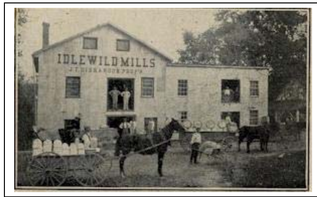
Idlewylde Mills at Federalsburg.
