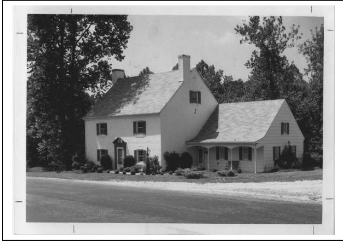
Knotts Mill converted to dwelling, 1970 photo by Michael Bourne.
