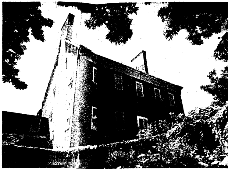
A rear view of the house, which stands at Prince George and East streets. The chimneys tower 90 feet above the ground.
