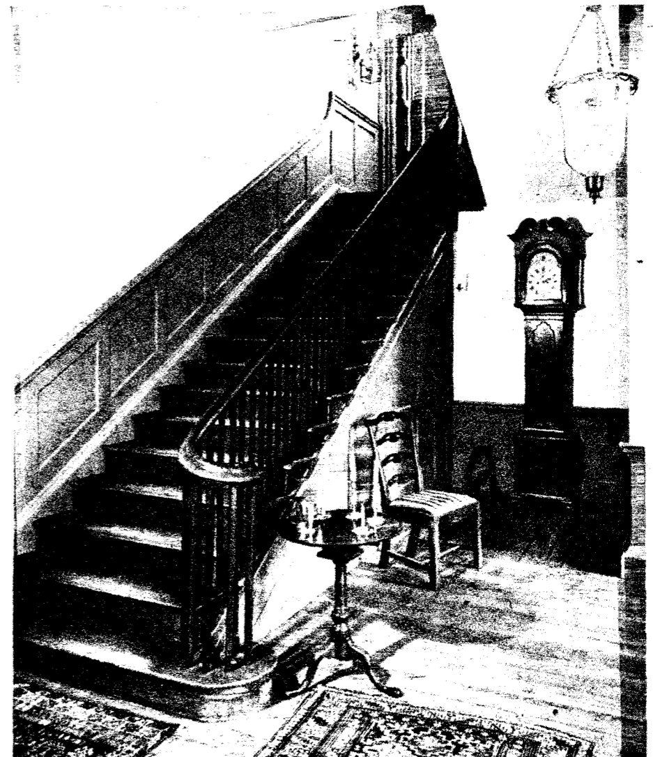
The stairway is Santo Domingo mahogany. Because the house had never been mutilated, Mrs. Wohl regards her work as "rejuvenation."
