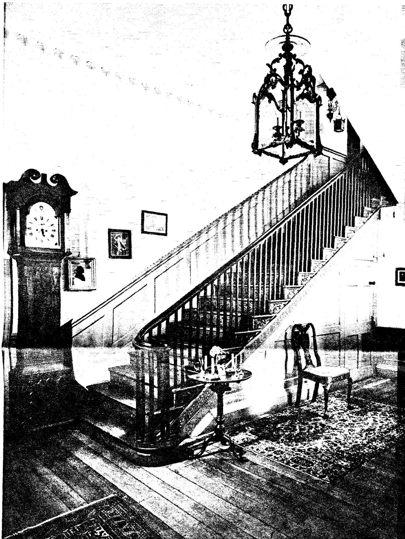
Santo Domingan mahogany staircase, with relief carved step ends and grooved balustrade, is an example of the Colonial craftsmanship in the 200-year-old house.
