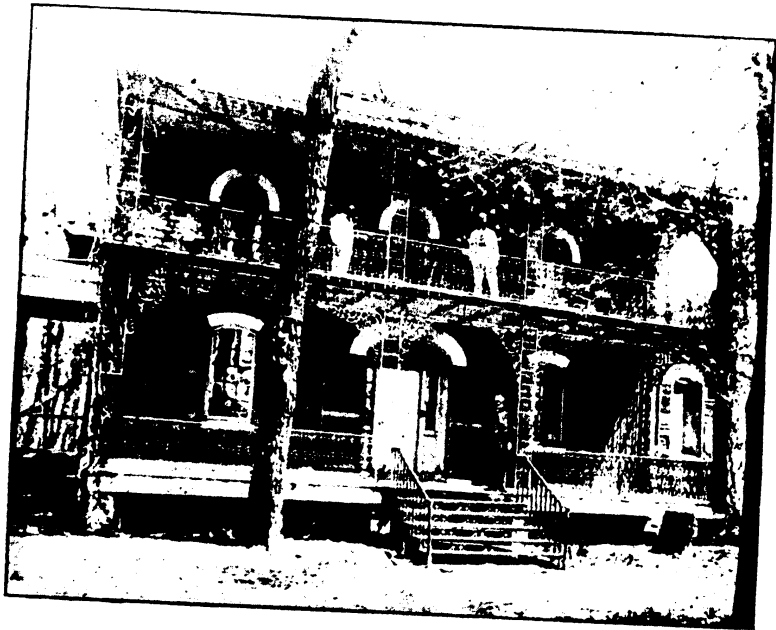
THE SUPERINTENDENT'S HOUSE.
