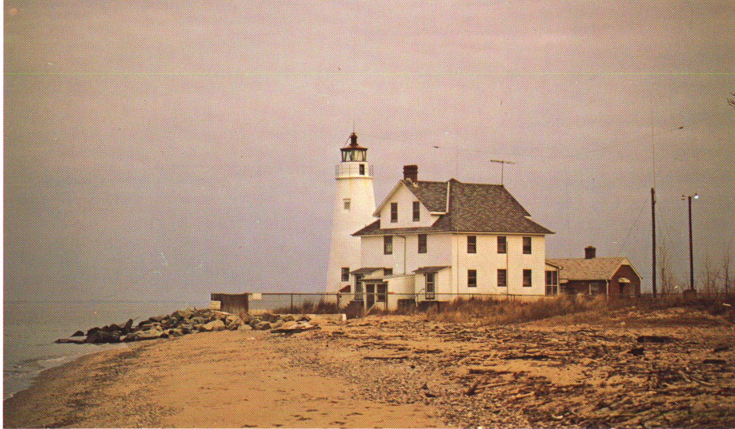
COVE POINT LIGHTHOUSE, CALVERT COUNTY
