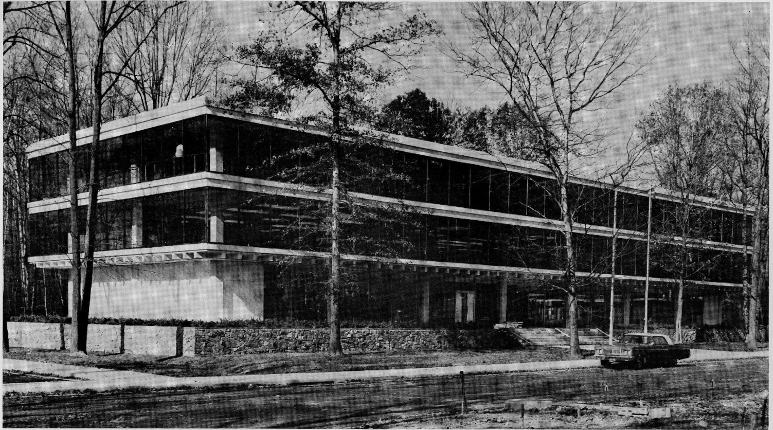
PRINCE GEORGE'S COUNTY REGIONAL HEADQUARTERS, MARYLAND-NATIONAL CAPITAL PARK AND PLANNING COMMISSION, RIVERDALE
