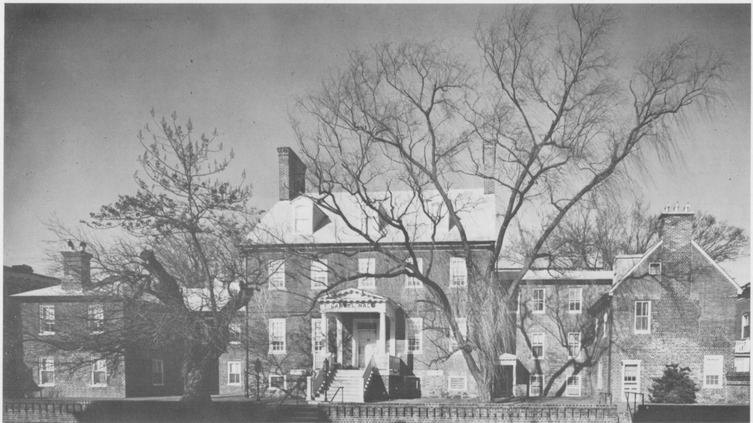
PACA HOUSE, ANNAPOLIS Photograph by M. E. Warren
