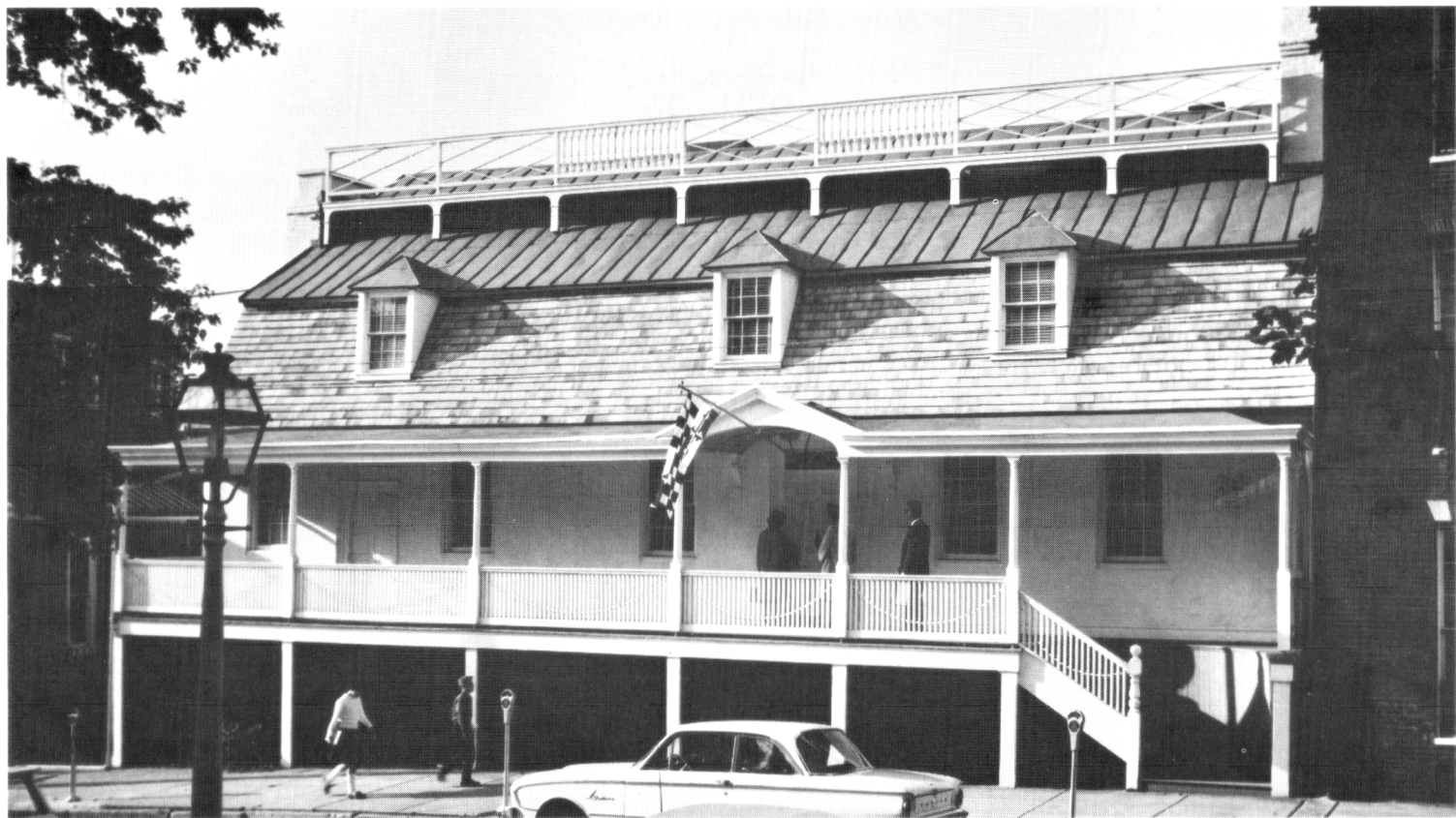
SHAW HOUSE, ANNAPOLIS. HOUSE OF DELEGATES ANNEX
