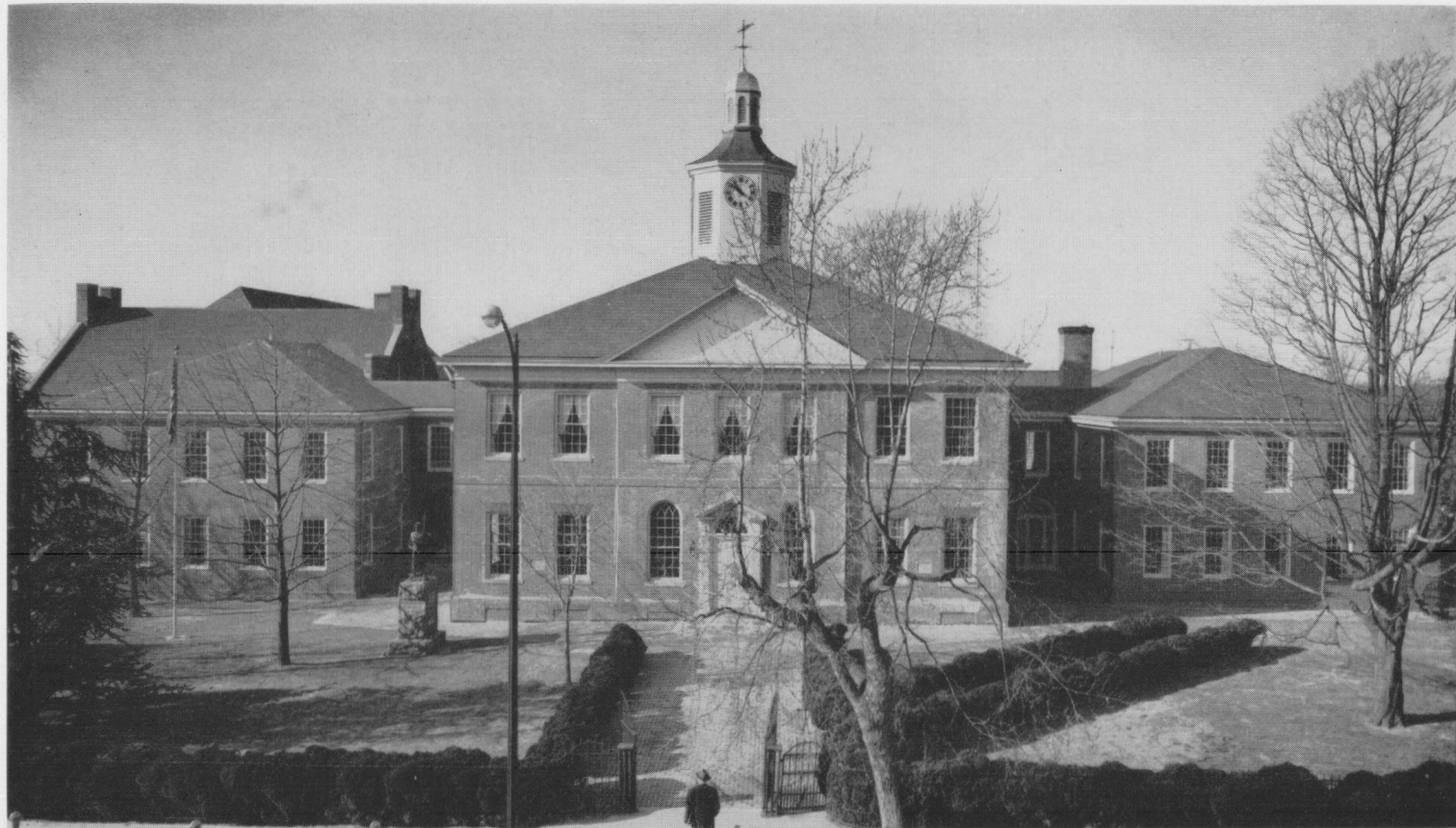
TALBOT COUNTY COURTHOUSE ADDITIONS, 1958 Easton
