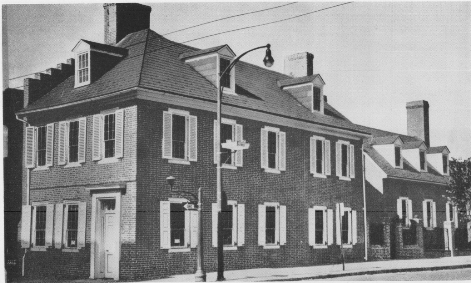
STAR SPANGLED BANNER FLAG HOUSE AND MUSEUM BUILDING RESTORATION Baltimore
