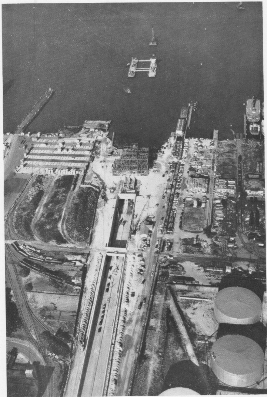
FAIRFIELD PORTAL BALTIMORE HARBOR TUNNEL Completed 1957
