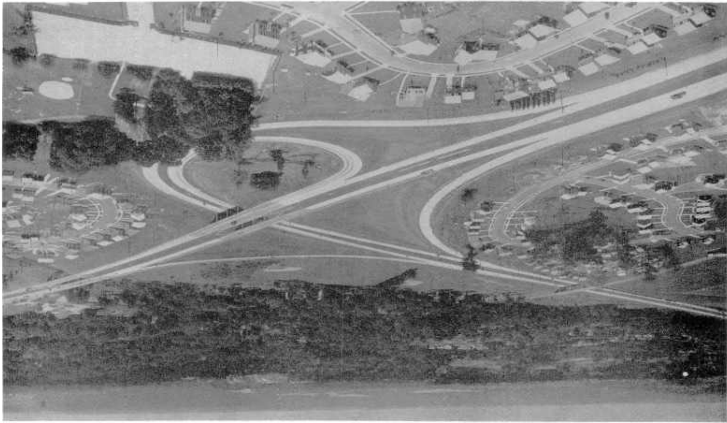
INTERCHANGE—BALTIMORE BELTWAY AND HARRISBURG EXPRESSWAY Courtesy of the Bureau of Highway Information, State Roads Commission
