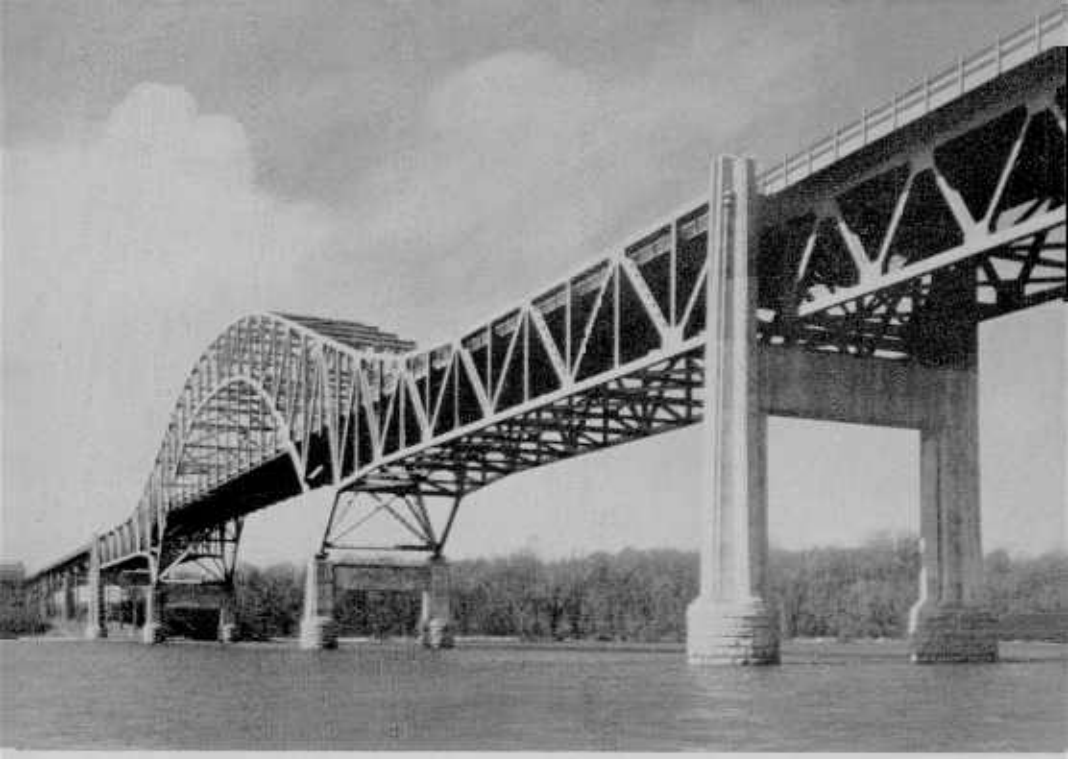
SUSQUEHANNA RIVER BRIDGE U. S. ROUTE 40 ↓
