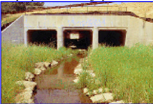
New stream crossing with reconstructed trout habitat at Owings Mills New Town
