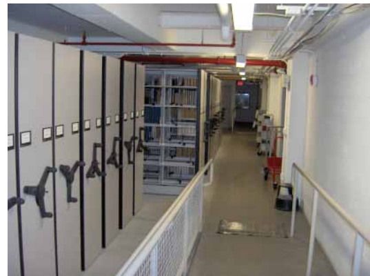
Mobile Shelving Chemical Heritage Foundation
