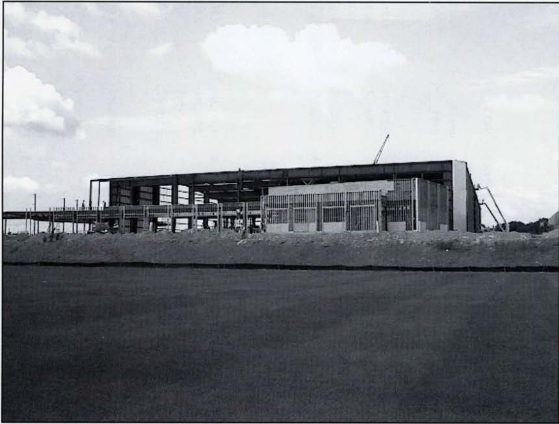
New construction at the South Germantown Recreational Park includes the SoccerPlex indoor soccer facility, outdoor stadium, soccer fields and much more.
