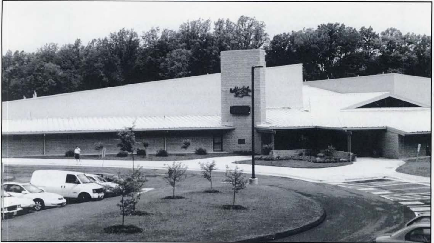
The new Cabin John Ice Rink features three indoor rinks, a warming room, team room, concession area, arcade and offices.
