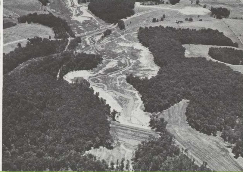
An aerial photo taken on July 1, 1965 reveals the completion of the dam and its spillway and the outline—dramatically formed by trees—of what will be a 74-acre permanent lake. Once filling begins, it will take the water about a year to reach its permanent level.
