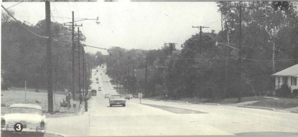
(3) River Road near Little Falls Branch Parkway.
