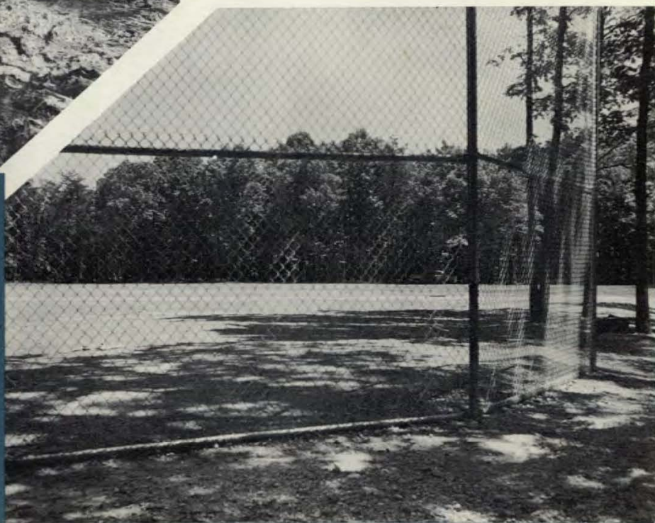
A major program in the southern Prince George's County portion of the park district last year was the development of the 26-acre Bradbury Recreation Center near Bradbury Heights. The aerial view shows the access roads to and from the parking area and athletic field. The two photos show the extent of clearing which had to be undertaken to provide an athletic field.
